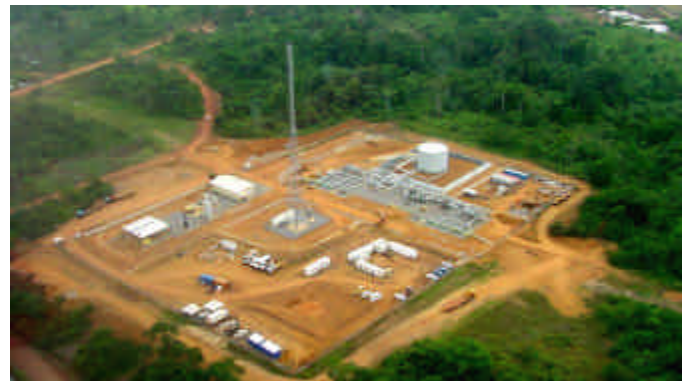
Figure 3C. Aerial view of the Pressure Reducing Station near Kribi, Cameroon.
