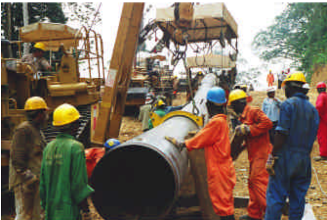
Figure 3A. Construction of the export pipeline.
