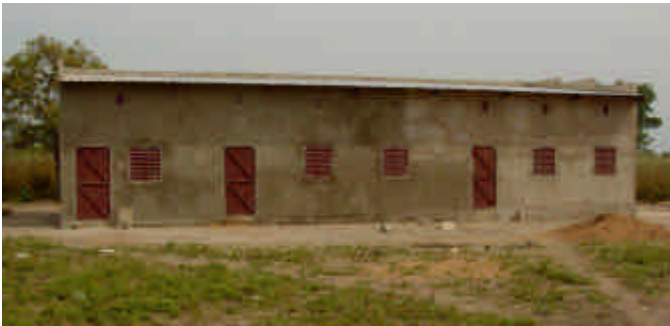
Figure 10C. A new classroom building built in the village of Begon I as part of the Project's community compensation program in Chad.
