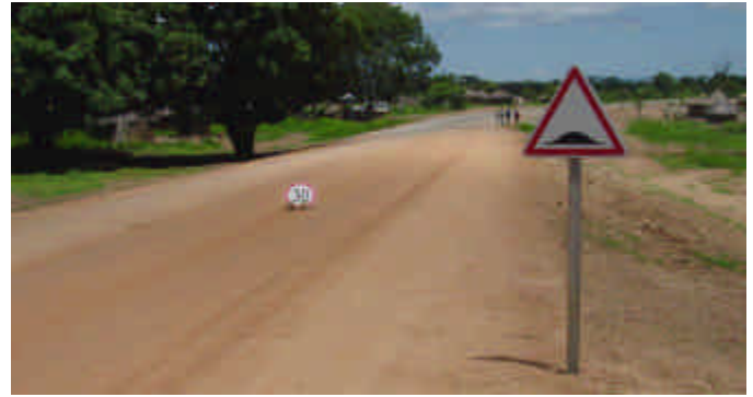
Figure 4C. A Project-upgraded road in northeastern Cameroon.
