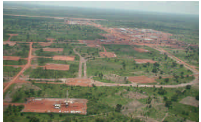
Figure 2A. Aerial view of a portion of the Komé oilfield area showing drilling pads and the CTF. An active drilling rig appears in the foreground.
