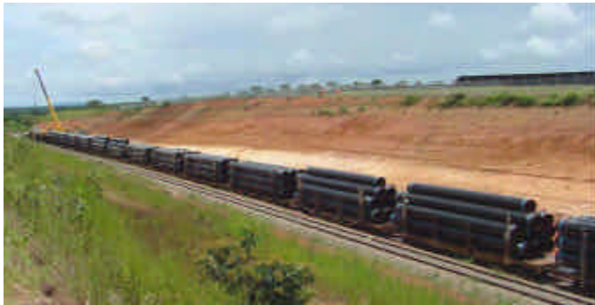
Figure 4A. Project-upgraded rail cars laden with pipes destined for storage yards.
