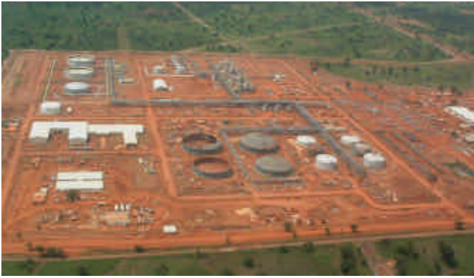
Figure 2B. Aerial view of the CTF. The four power generation units and Pump Station #1 are in the upper middle portion of the photograph.
