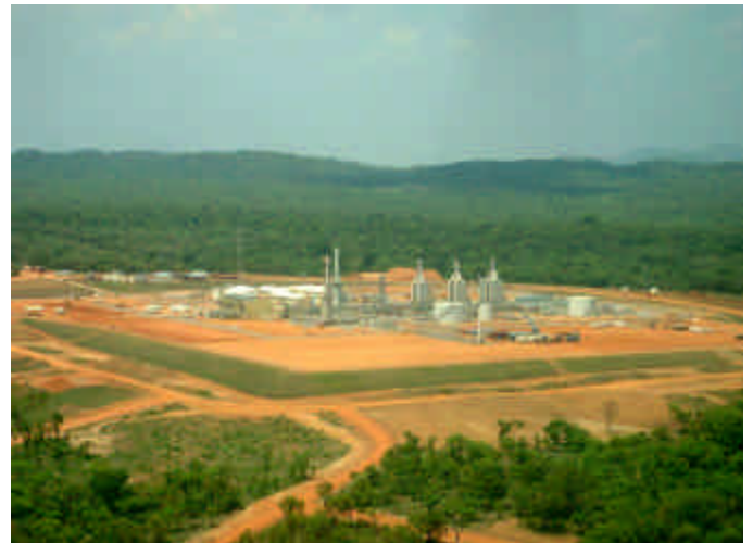
Figure 3B. Aerial view of Pump Station #2 near Dompta, Cameroon.
